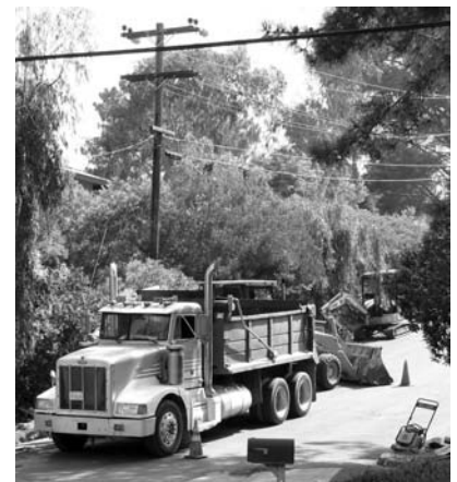
Undergrounding under way on Camino del Mar
